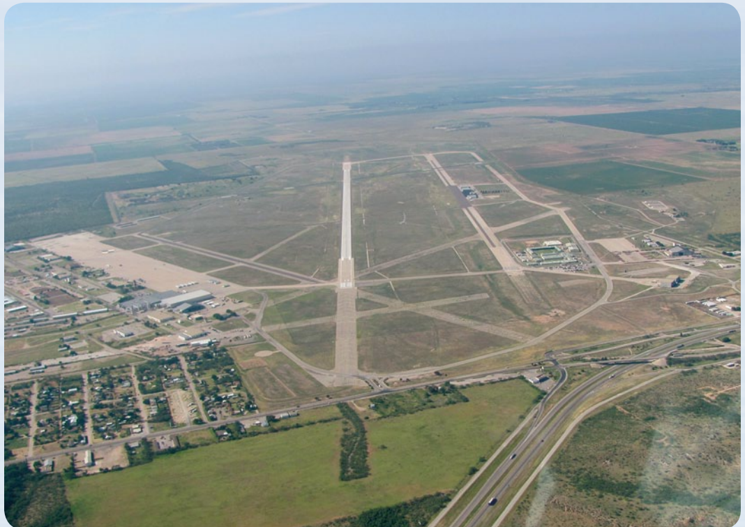
The newly reconstructed runway (17-35) is visible in this aerial photo of Big Spring McMahon-Wrinkle Airport. Special thanks to Marc Marchesseault for the airplane ride.
