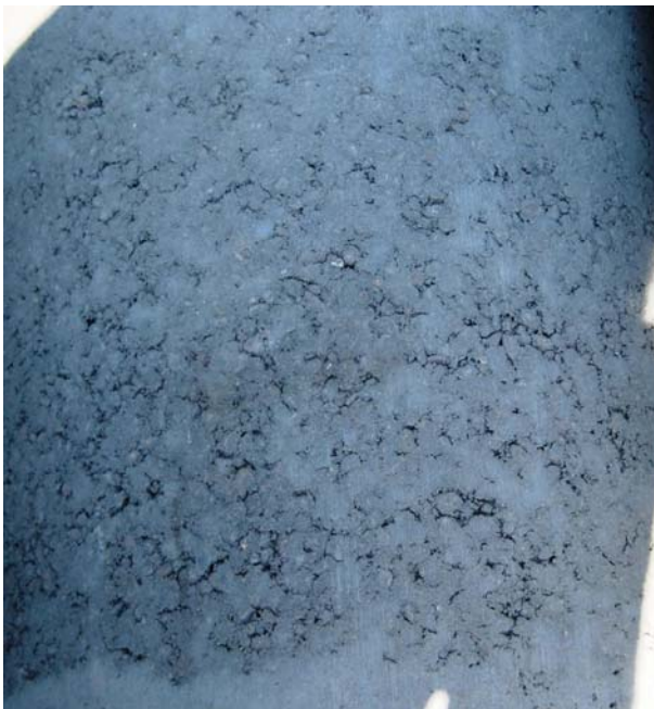
Figure 60-2—Honeycombed Concrete.
