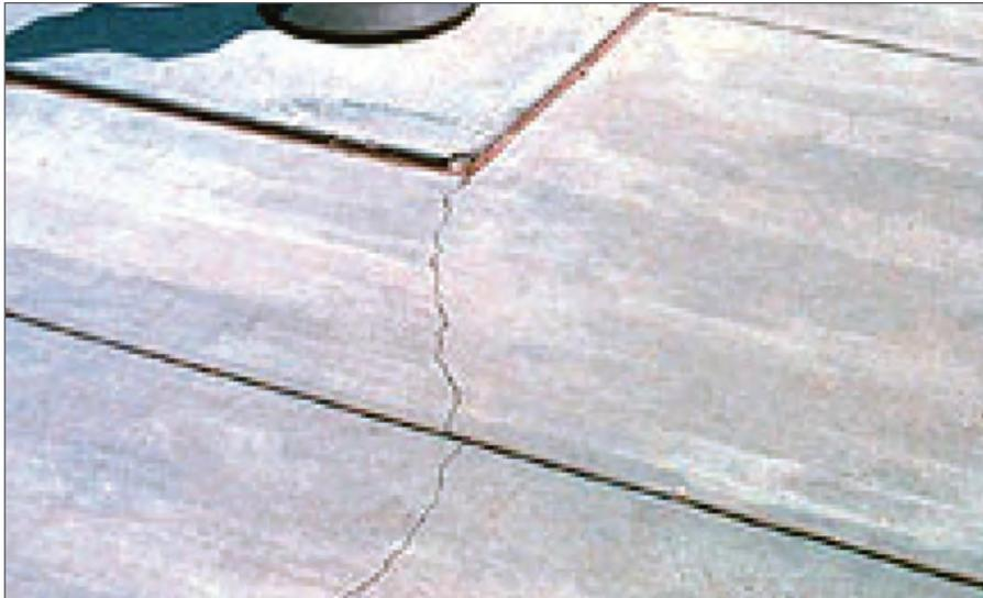
Figure 3. Drying Shrinkage Cracking.
