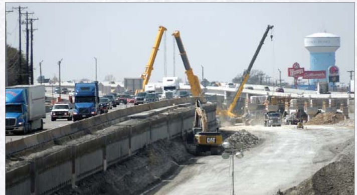
LBJ Express construction at Midway Road looking west.
