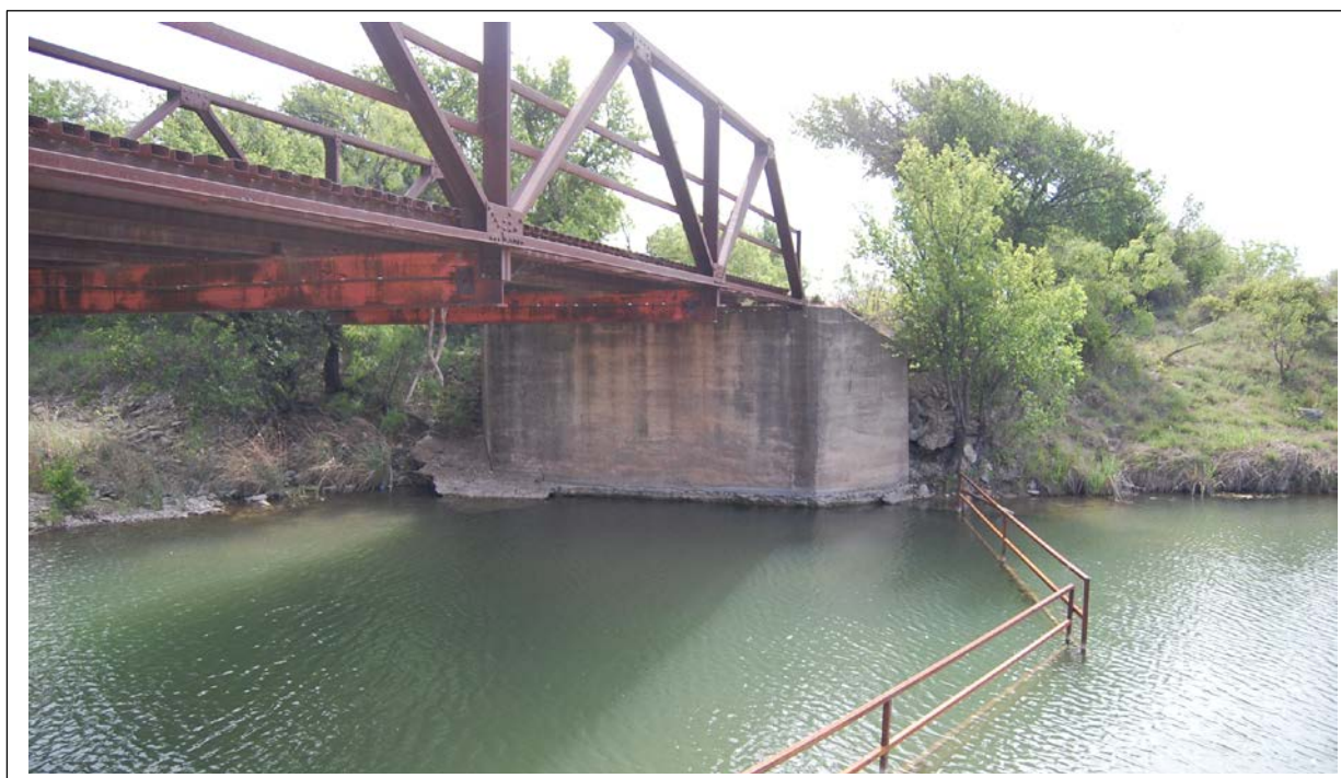
Photo taken from south side of structure facing east.
