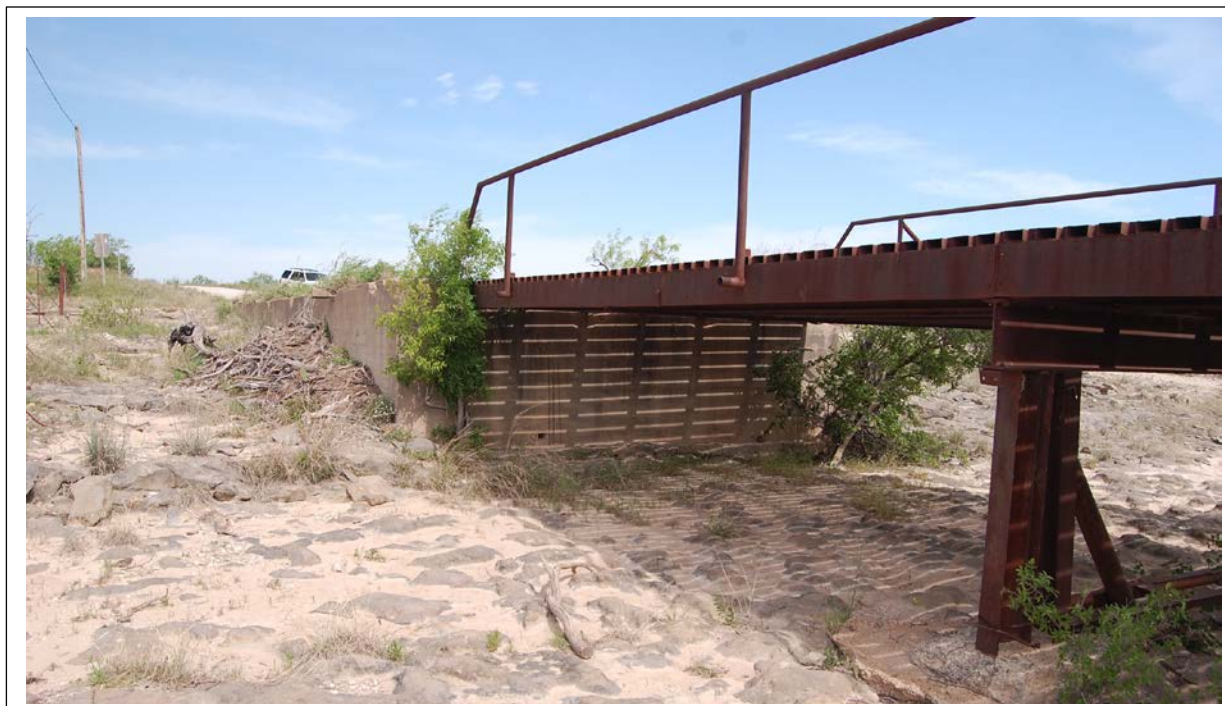
Photo taken from south side of structure facing west.
