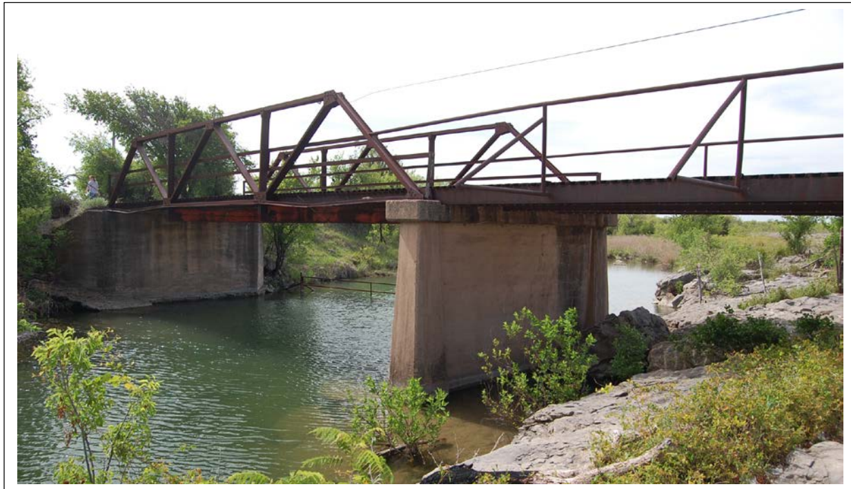
Photo taken from north side of structure facing east.
