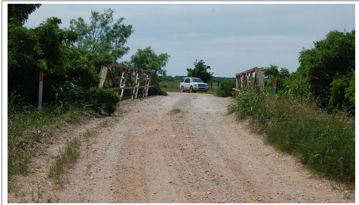
Photo taken from the east side of the structure.
