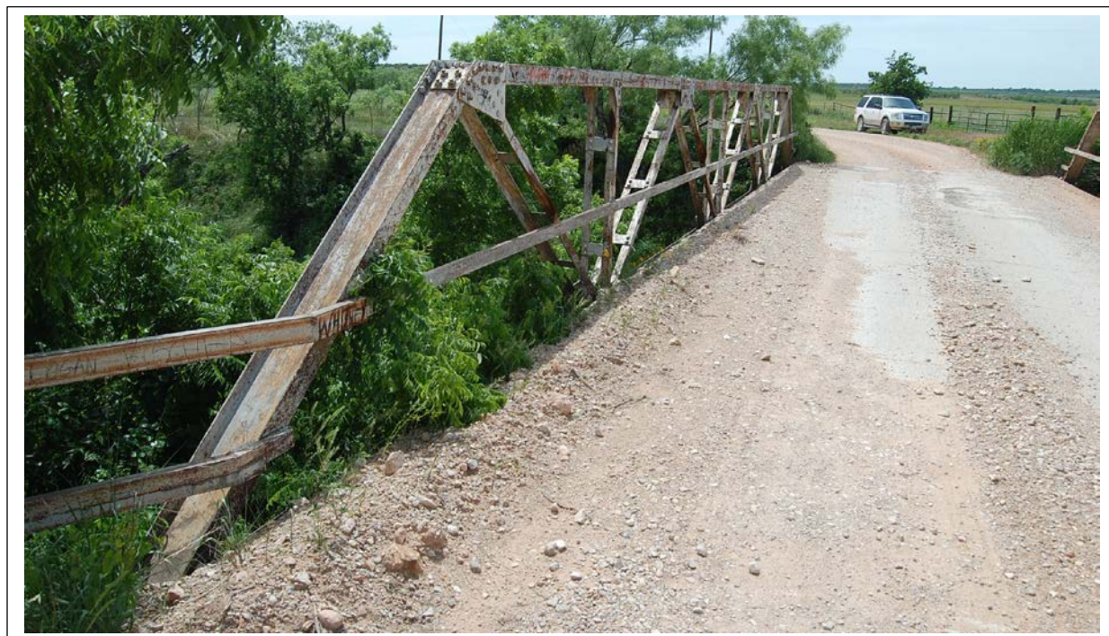
Photo taken from east side of the structure facing westward.
