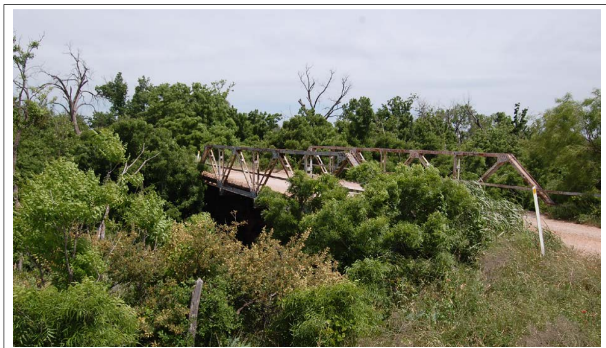
Photo taken from the northwestern side of the structure.
