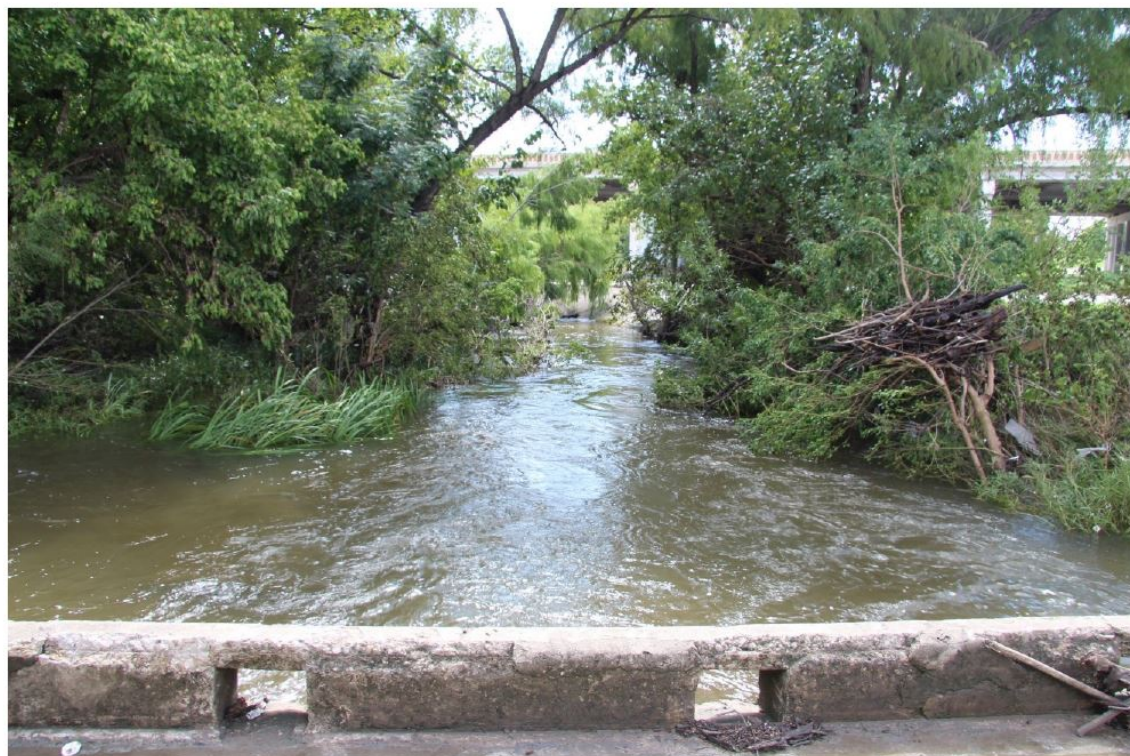
View facing southeast, showing Cibolo Creek downstream channel. IH 35 in background.
