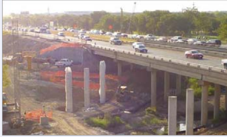
Fall 2011 -- I-820 bridge work at Big Fossil Creek
