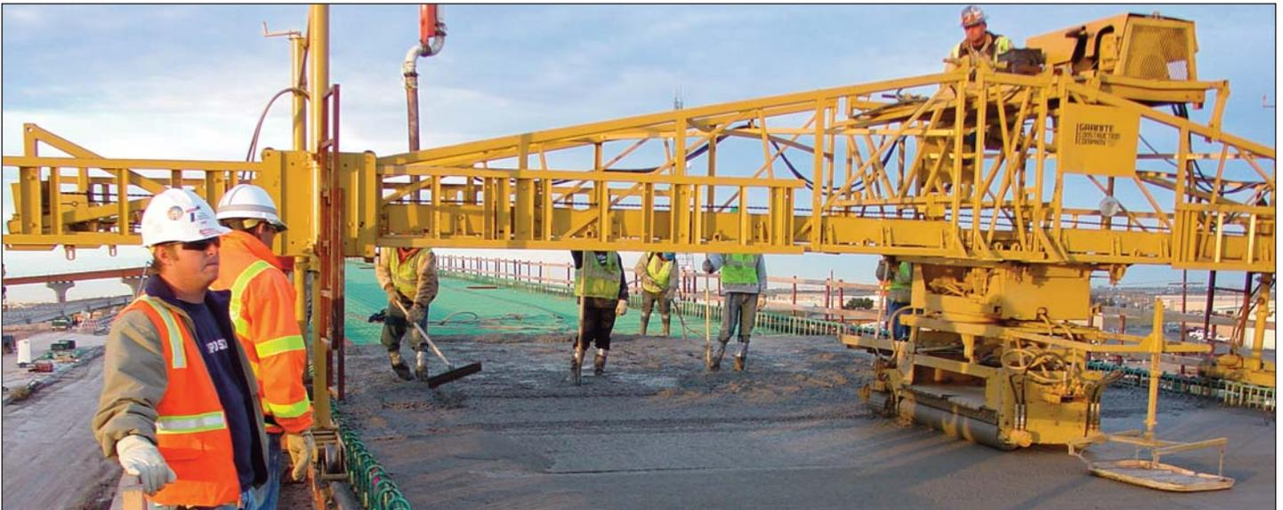
Contractors pour concrete to form a portion of the bridge deck on the 3,900-foot flyover at West Loop 289 and Brownfield Highway. Construction of the flyover is part of Phase 3A of the Marsha Sharp Freeway project. This phase will complete this fall.
