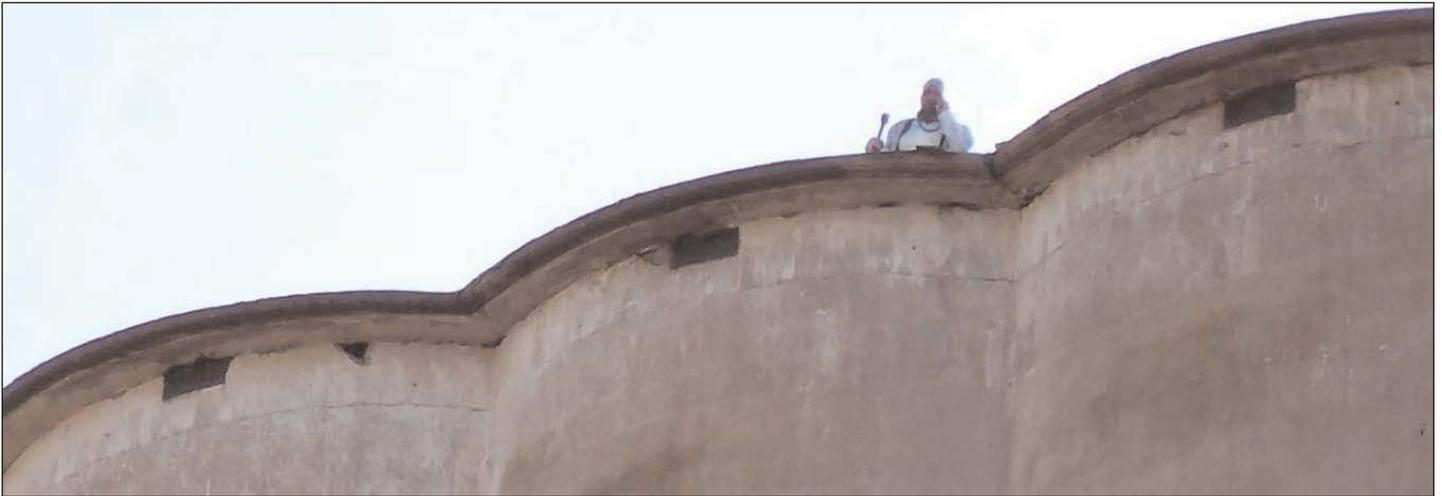
A worker removes asbestos material from the top of the Burrus Elevator. The contractor is required to abate the asbestos before the elevator can be demolished.
