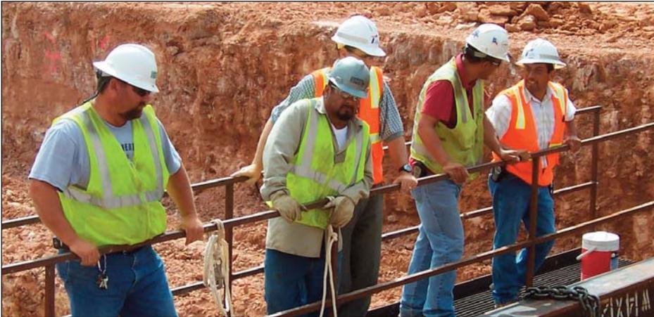
Granite and TxDOT employees look on as a concrete drainage conduit is lowered into the the ground on Phase 2 of the freeway project. Below, a Granite employee seals the joints between the conduits.
