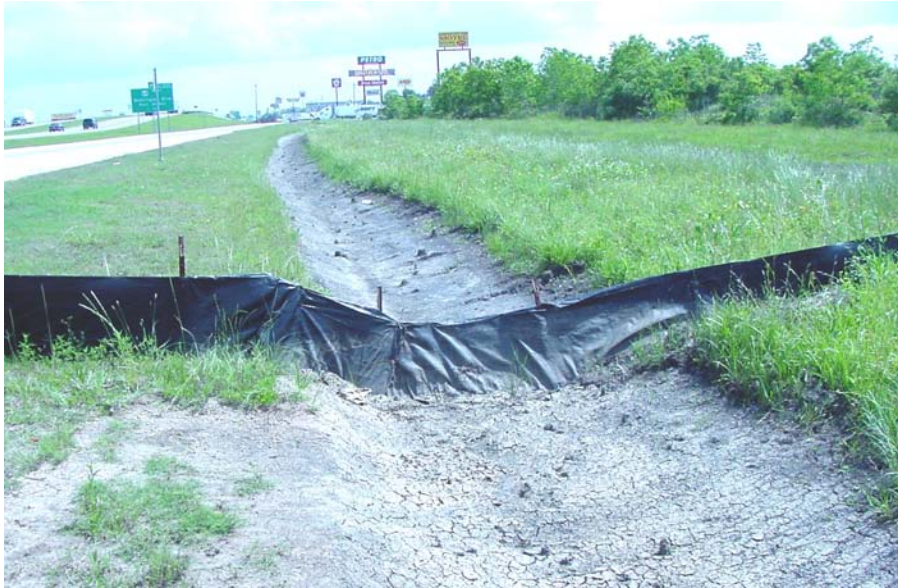
Figure 2.3 - Example of limiting disturbed area. Note the extent of vegetation left in place.
