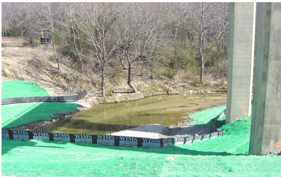
Figure 4.5 – Soil retention blankets used, in conjunction with silt fence, to stabilize a slope.
