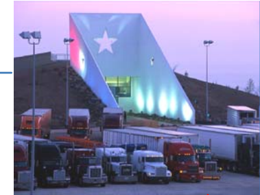
"Earth-Shelter" design of the Gray County (IH-40, east of Amarillo) facility emulates natural rock outcroppings common in the area while conserving building thermal energy.
