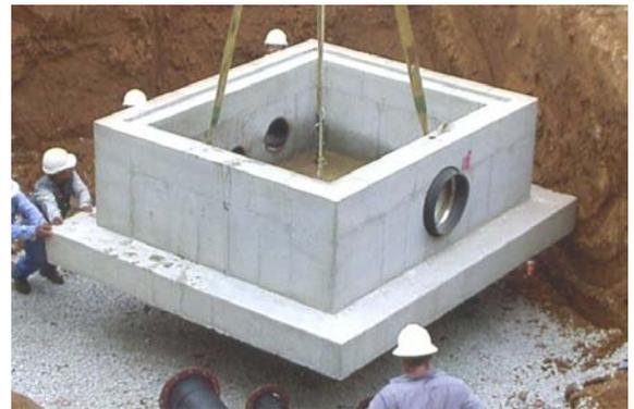
Figure 5: Leveling Course of Select Granular Material
