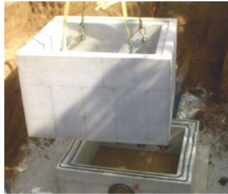
Figure 7: Gasket Material Installed on Top and Bottom of Joint Shoulders
