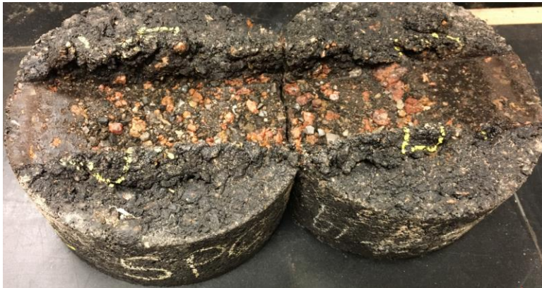
Figure 4 —Example of Visibly Stripped Aggregate in Hamburg Sample
