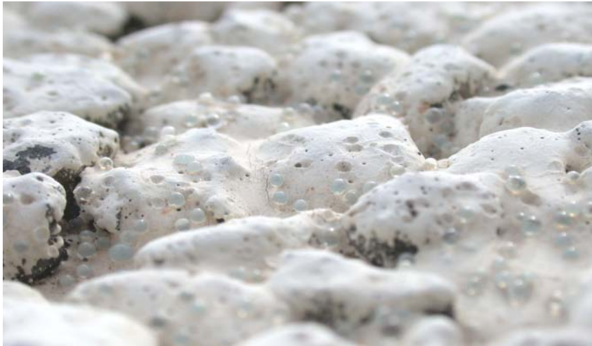
Figure 6. Thin-line thermoplastic application showing bead loss
