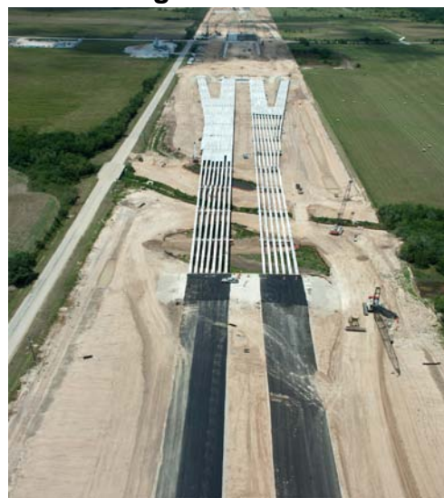
SH 99 Segment E Bear Creek
