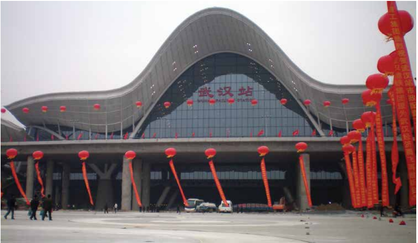
Wuhan Railway Station, Wuhan, China
