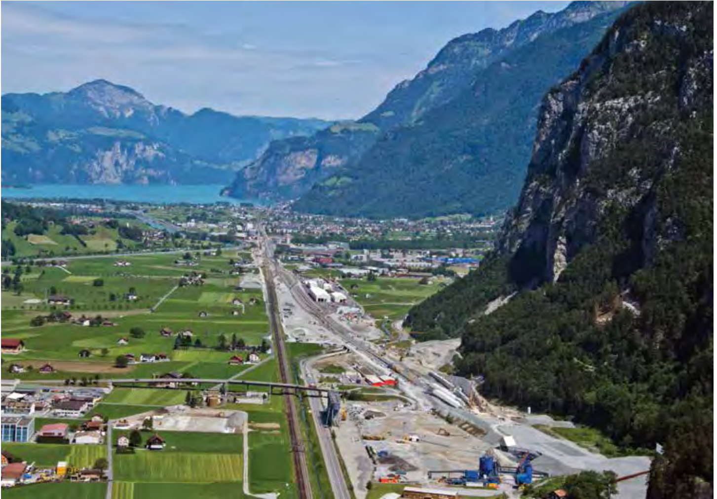
Gotthard Base Tunnel Project near Ersfeld ©Gotthard
