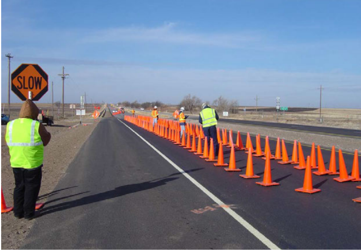
Figure 3. Typical External Survey Station.
