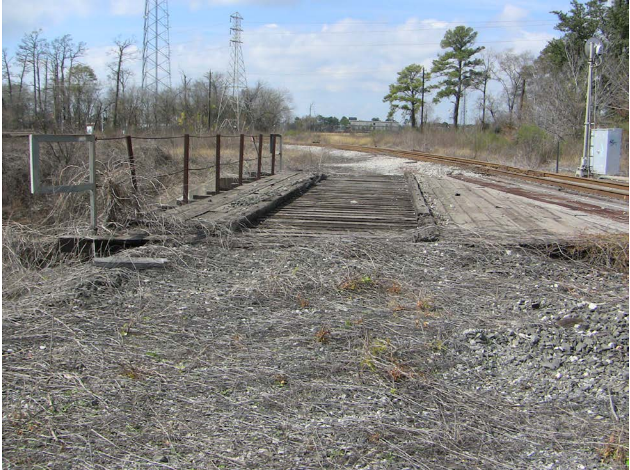
Existing Middle bridge looking west.
