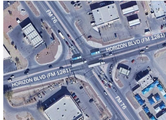
Figure 8: FM 76 and Horizon Blvd (FM 1281) Intersection
