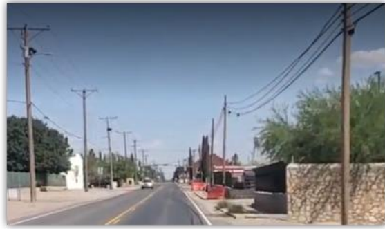
Figure 2: FM 76 (North Loop Dr) Near the End of the Corridor
