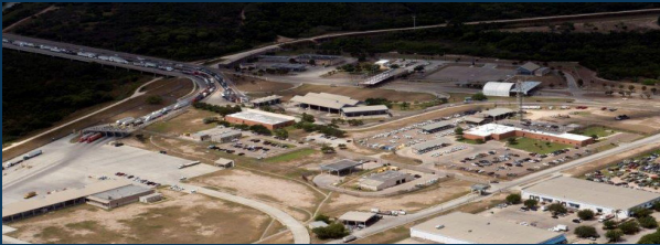
Veterans International Bridge at Los Tomates Port-of-Entry (POE)
