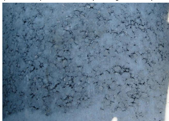
Figure 59-2. Honeycombed concrete
