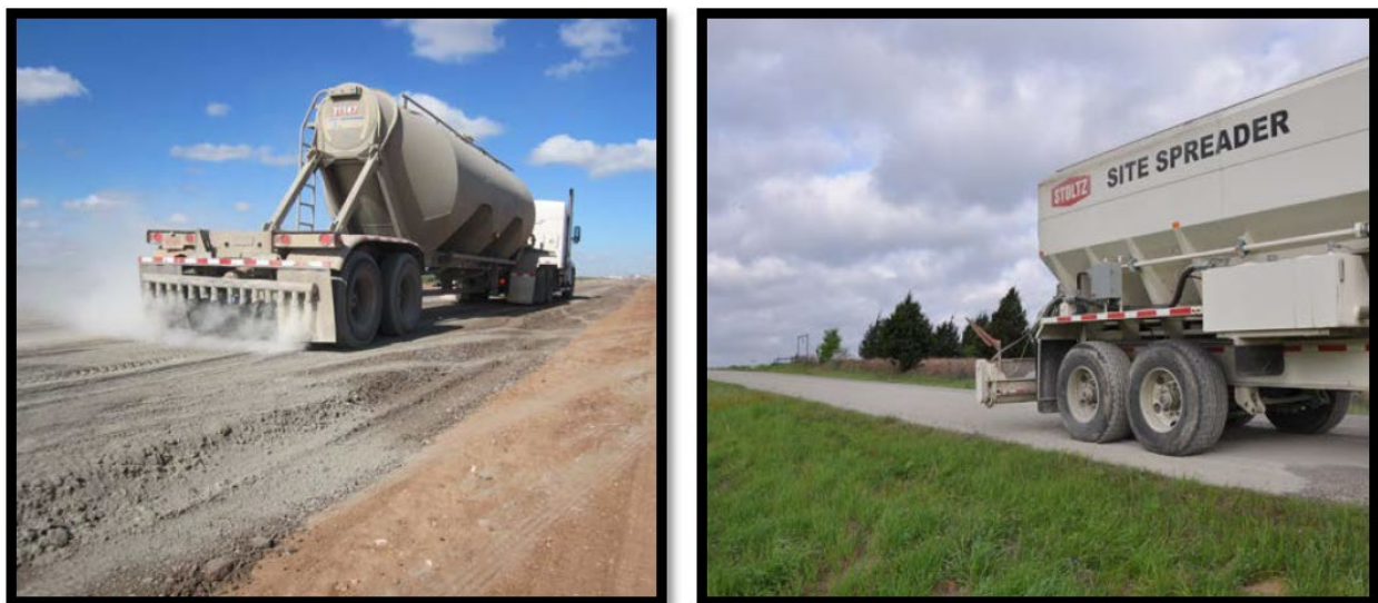
Figure 3 - Blown (Left) and Spread (Right) Cement Application.
