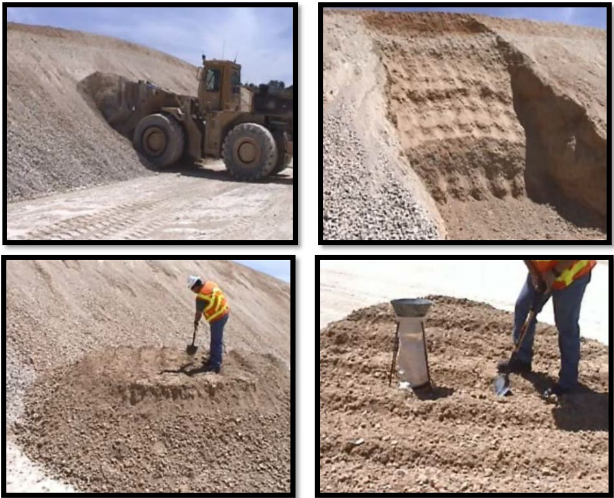
Figure 8 - Sampling a Stockpile of Flexible Base.
